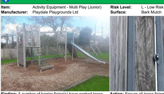
Finding: A number of barrier fixing(s) have worked loose
