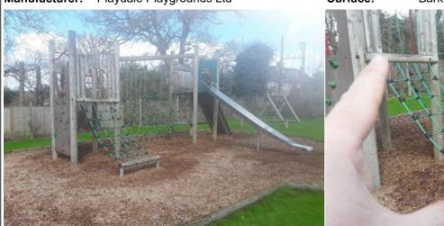
Finding: The net anchor timber forms a hard object within the falling space of the equipment in contravention of the requirements of BS EN 1176 Part 1
