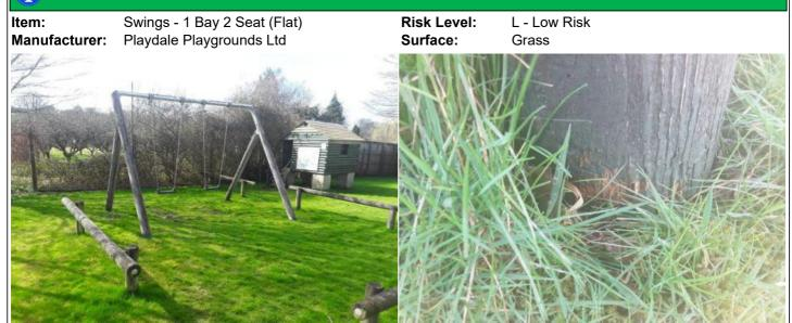
**Finding:** There is some strimmer / machinery damage apparent on the posts, this can penetrate the preservative applied to the timber and accelerate the rotting process
