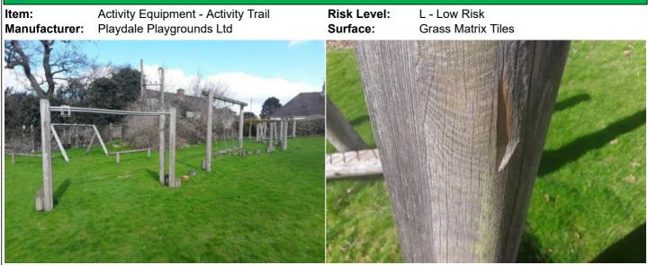
Finding: Parts of the timber are rough or splintered
