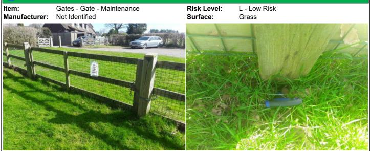
**Finding:** There are areas or parts of the timber on the structure that have rotted
