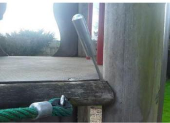
Finding: There is/are finger entrapment/s between platform Action: Monitor - No remedial work recommended and post and the item fails to meet the requirements of BS EN 1176 Part 1 4.2.7.6 Entrapment of fingers
