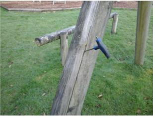
Finding: The timber has a number of air cracks apparent, the splits will have penetrated the preservative applied to the timber and allow water ingress to the unprotected areas
