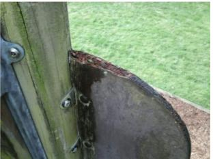
Remove all rough or splintered edges. Finding: The plywood has delaminated in some places Action:
