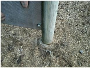
Finding: The surface has eroded and the foundations are exposed
