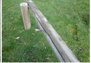
The timber has a number of air cracks apparent, the splits will have penetrated the preservative applied to the timber and allow Finding: water ingress to the unprotected areas
