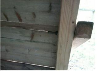
Action: Remove excess thread length and deburr or Finding: There are projecting bolt thread(s) present
