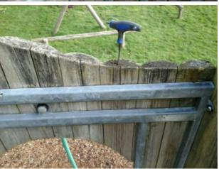
Finding: There is some evidence of rot in the timber of Action: the barrier by the pull up rope
