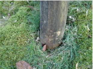
Finding: There is some strimmer damage apparent on Action: the posts, this can penetrate the preservative applied to the timber and accelerate the
