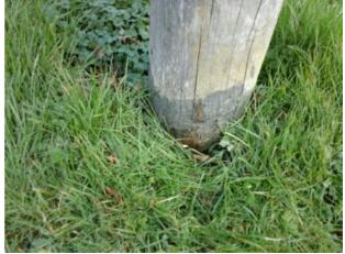
There is some strimmer damage apparent on the posts, this can penetrate the preservative applied to the timber and accelerate the Finding:
