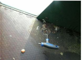
The plywood has delaminated in the deck by Action: the slide Finding:
