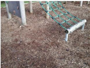
Finding: The level of loose fill surfacing has fallen significantly below the minimum 200mm recommended by BS EN 1176 Part 1
