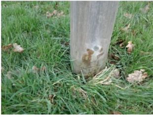
There is some strimmer damage apparent on the posts, this can penetrate the preservative applied to the timber and accelerate the Finding:
