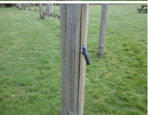
Finding: The timber has a number of air cracks
