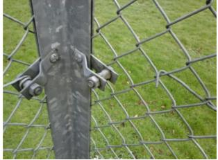
Finding: Fixings are damaged and/or have sharp edges
