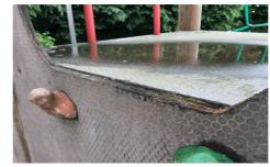
Task: Rub down and treat damaged edges
