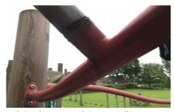
Task: De-scale and coat with lead free paint, using appropriate precautions
