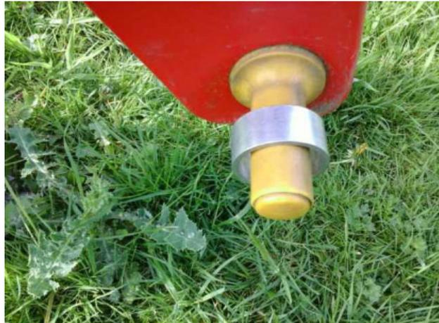
**Finding:** The end of handgrips and/or footrests have a cross section of less than 15cm<sup>2</sup> and fail to meet the requirements of BS EN 1176:2008 Part 6
