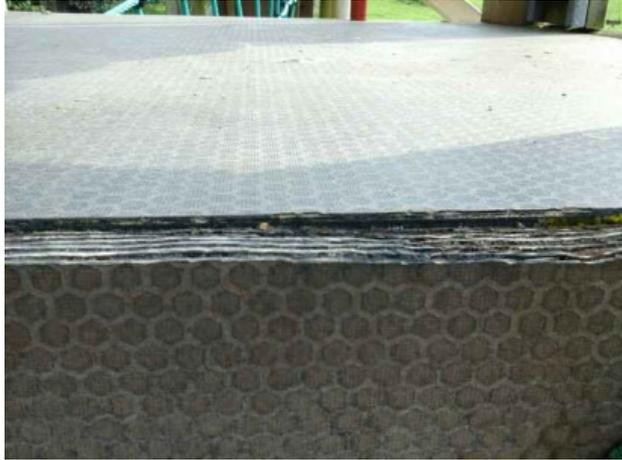
**Finding:** Parts of the timber are rough or splintered **Action:** Remove all rough or sharp edges
