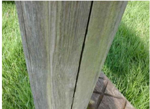
**Finding:** The timber has a number of air cracks apparent, the splits will have penetrated the preservative applied to the timber and allow water ingress to the unprotected areas
