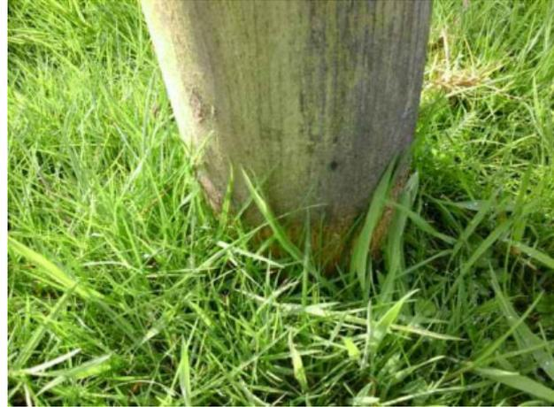
**Finding:** There is some strimmer damage apparent on the posts, this can penetrate the preservative applied to the timber and accelerate the rotting process
