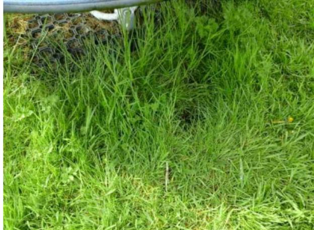
**Finding:** The grass mats are silted up, the soil is compacted and the area will become very slippery when the soil is wet.
