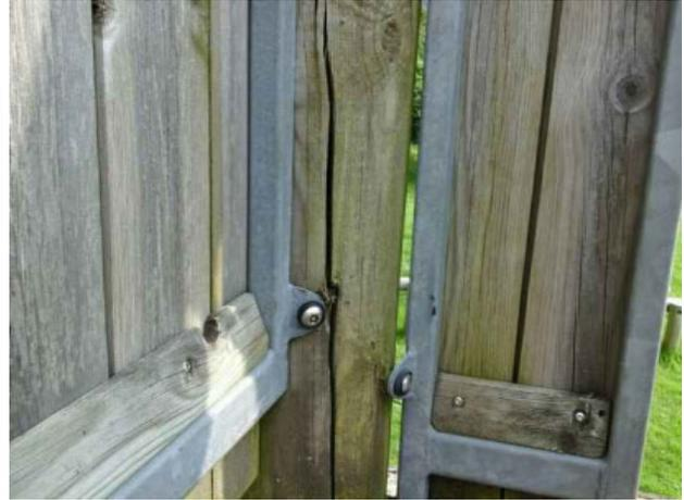
**Finding:** A number of fixing(s) have worked loose on the barriers **Action:** Secure all loose fixings
