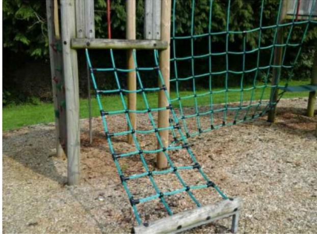
**Finding:** The lower timber forms a hard object within the falling space of the equipment in contravention of the requirements of BS EN 1176 Part 1
