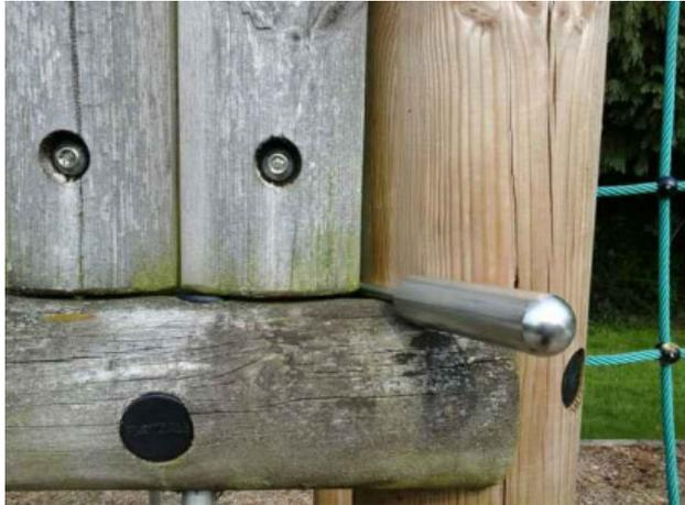
**Finding:** There is/are finger entrapment/s in the barrier corners and the item fails to meet the requirements of BS EN 1176:2008 Part 1 4.2.7.6 Entrapment of fingers **Action:** Monitor use
