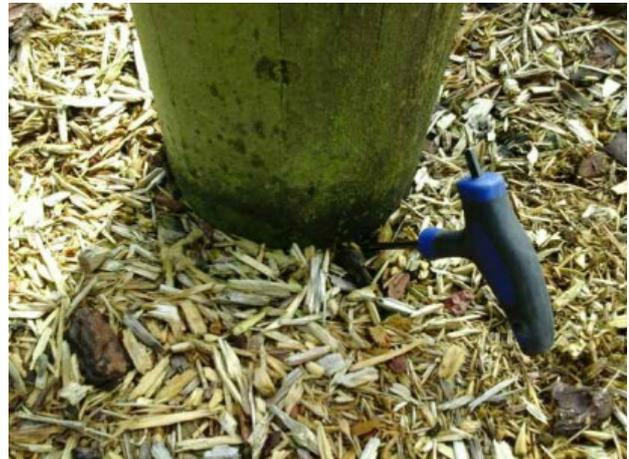
**Finding:** There is some evidence of rot in the timber **Action:** Monitor for any further deterioration and replace as required
