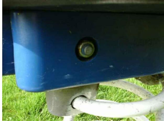
**Finding:** There is/are bolt cap covers missing or damaged on the item
