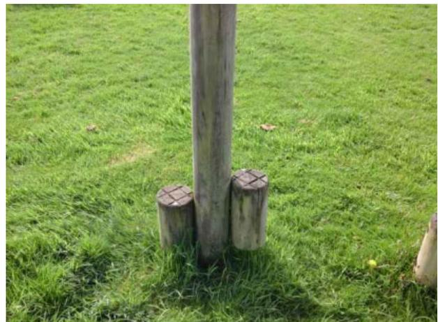
**Finding:** The item is slightly loose in its foundations on the stilts
