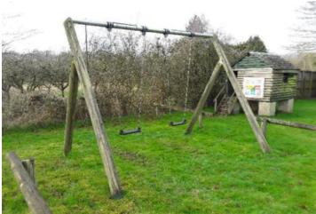
**Finding:** There is some strimmer / machinery damage apparent on the posts, this can penetrate the preservative applied to the timber and accelerate the rotting process
