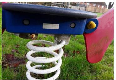
**Finding:** There is/are bolt cap covers missing or damaged
