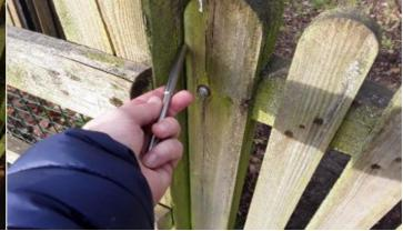
**Finding:** There are openings that are less than 12mm that could trap or crush fingers
