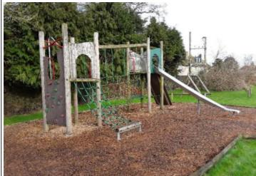
falling space of the equipment in contravention of the requirements of BS EN 1176 Part 1
