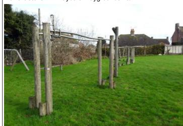
**Finding:** There is algae or moss on the surface of the equipment resulting in slippery conditions
