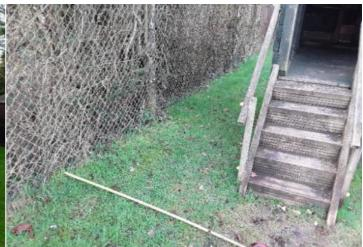
**Finding:** The fencing forms a hard object within the falling space of the equipment and there is also insufficient surfacing provided
