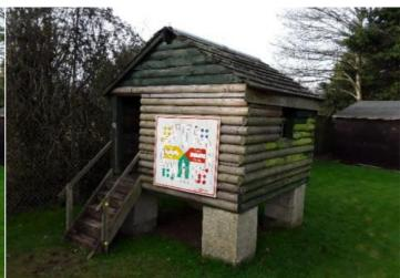
**Finding:** This equipment has not been designed or installed **Action:** Monitor use and review the use of the equipment to meet with the requirements of BS EN 1176 for public and risk assessment regularly
