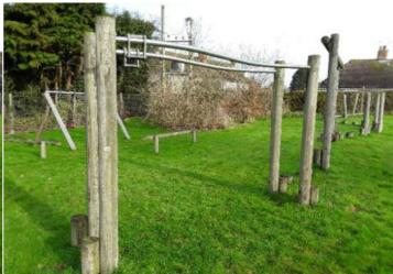
**Finding:** The item of equipment has a fall height exceeding **Action:** Monitor - no remedial action recommended 1.50 metres and grass has been provided as a safety
