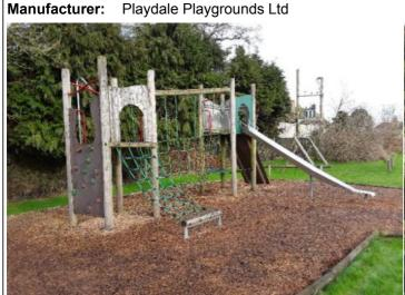
**Finding:** There is algae or moss on the surface of the equipment that can lead to the onset of rot
