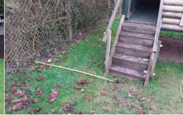
**Finding:** The fencing forms a hard object within the falling space / impact area of the equipment
