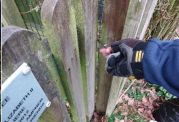
**Finding:** The opening between the gate and the post is less **Action:** Adjust gate to ensure a 12mm opening all around than 12mm and could trap users fingers
