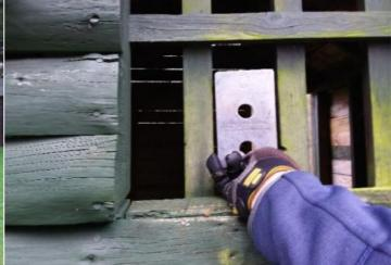
**Finding:** The item fails to meet the requirements of BS EN 1176 Part 1 4.2.7.2 for head and neck entrapment in the
