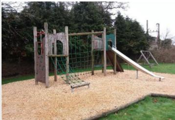
**Finding:** There is/are finger entrapment/s between barrier and post and the item fails to meet the requirements of BS EN 1176 Part 1 4.2.7.6 Entrapment of fingers
