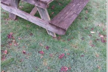
**Finding:** The table is not secured to the ground and there is **Action:** Secure the item to the ground some potential for the item to be moved within falling spaces of equipment
