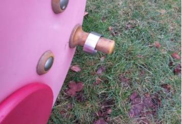
**Finding:** The end of handgrips and/or footrests have a cross **Action:** Monitor use section of less than 15cm2 and fail to meet the requirements of BS EN 1176 Part 6; this is however, a relatively low risk failure and no remedial action is recommended
