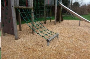
**Finding:** The base of the net forms a hard object within the **Action:** Monitor use falling space of the equipment in contravention of the
