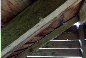
Finding: Parts of the timber are rough or splintered
